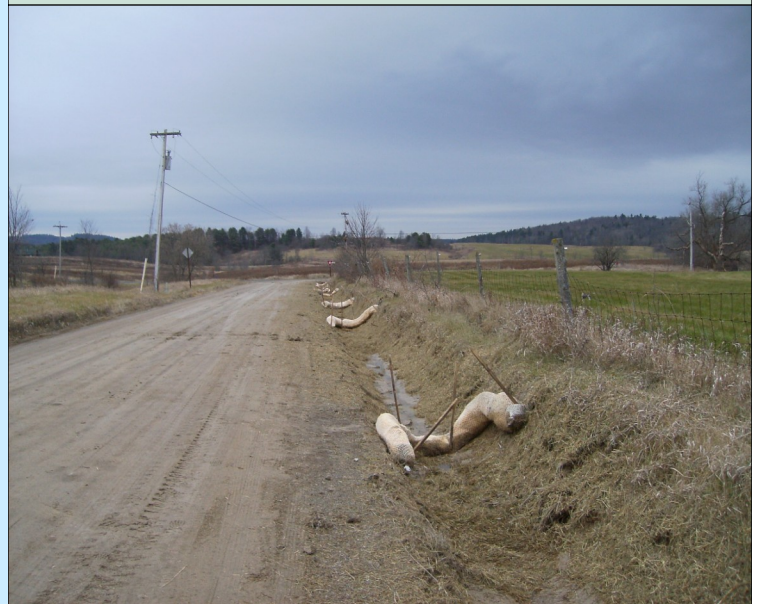
Example of a gravel road ditch erosion control sock check dams implemented in Essex County
