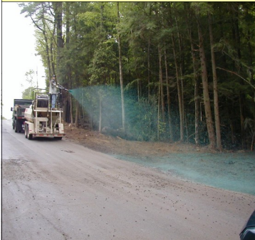
Road-Side Hydroseeding in Warren County
